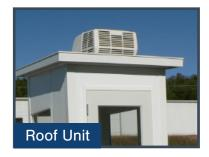
These units are similar to wall units, in that the air condenser and air handler are combined into one unit - however, the Coleman unit mounts on to the roof of the building. There is an air diffuser on the interior ceiling which also houses the controls for the unit unless the optional external thermostat is purchased. These units should only be used on flat roofs to avoid Condensation leaks.
